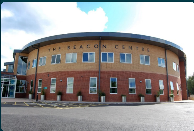
Figure 4 The Beacon Centre, Salford
